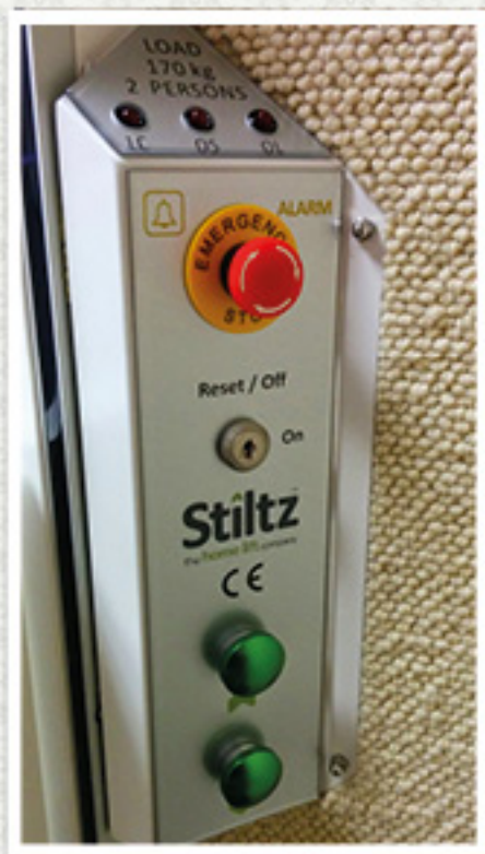
Stiltz Duo control panel
